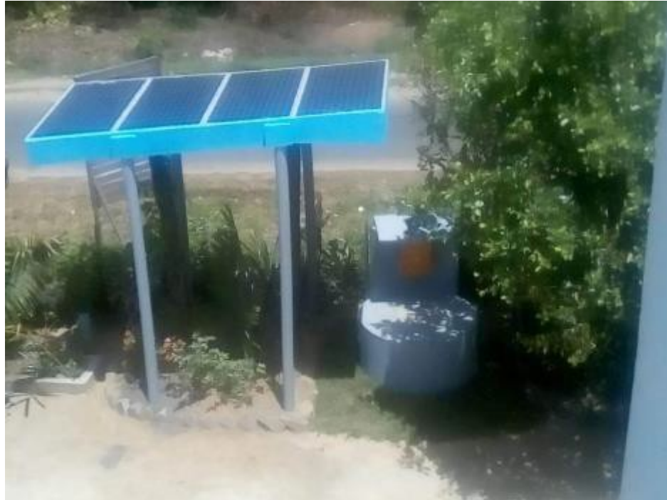
Well equipped with ferrocement nozzles - Support for ferrocement solar panel
