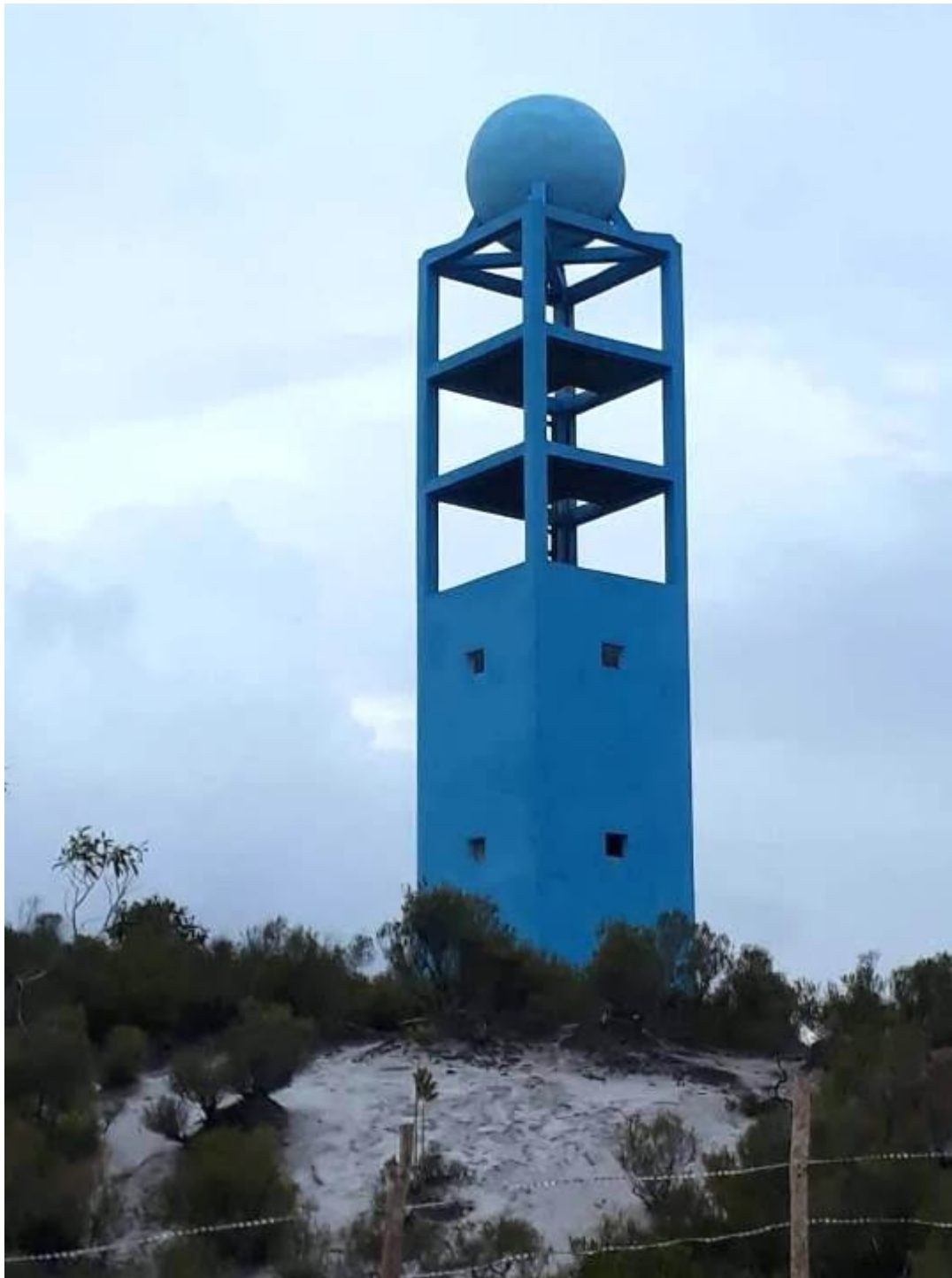
Ferrocement tank operating in a cyclonic zone and in a corrosive environment.
