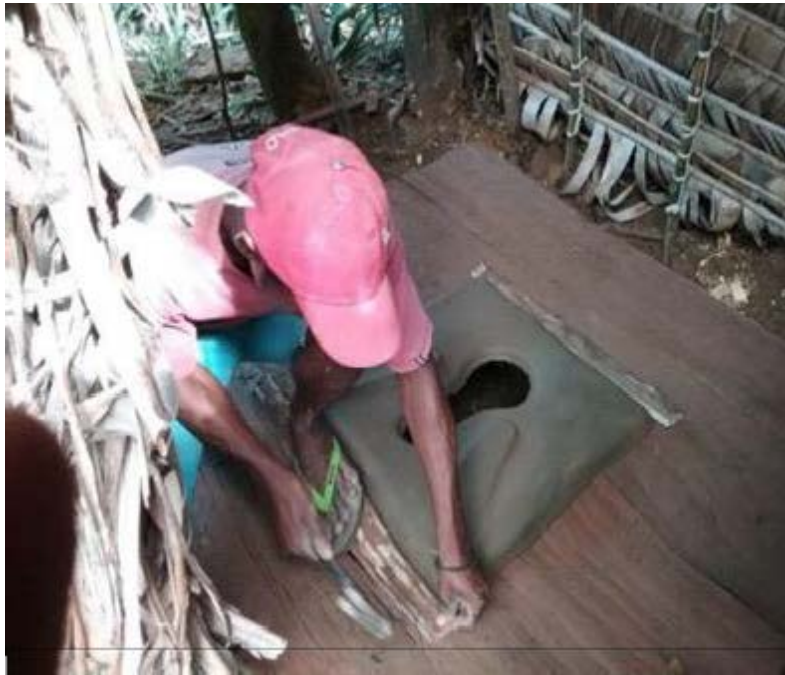
Local mason installing a SanPlat slab
