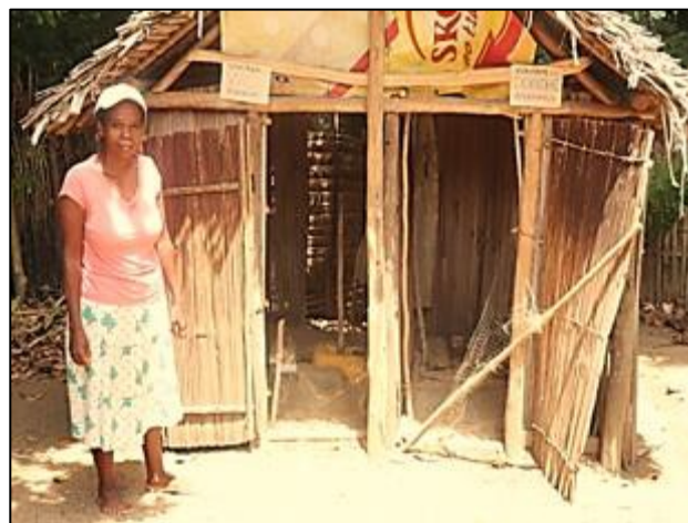
Honorine Vavisoa leads by example, installing a covered latrine and shower at her home.
