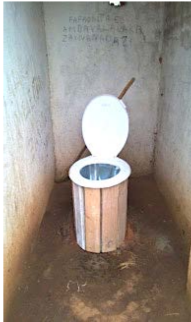
The latrine before and after the placement of the seat. (photo credit RANO WASH)
