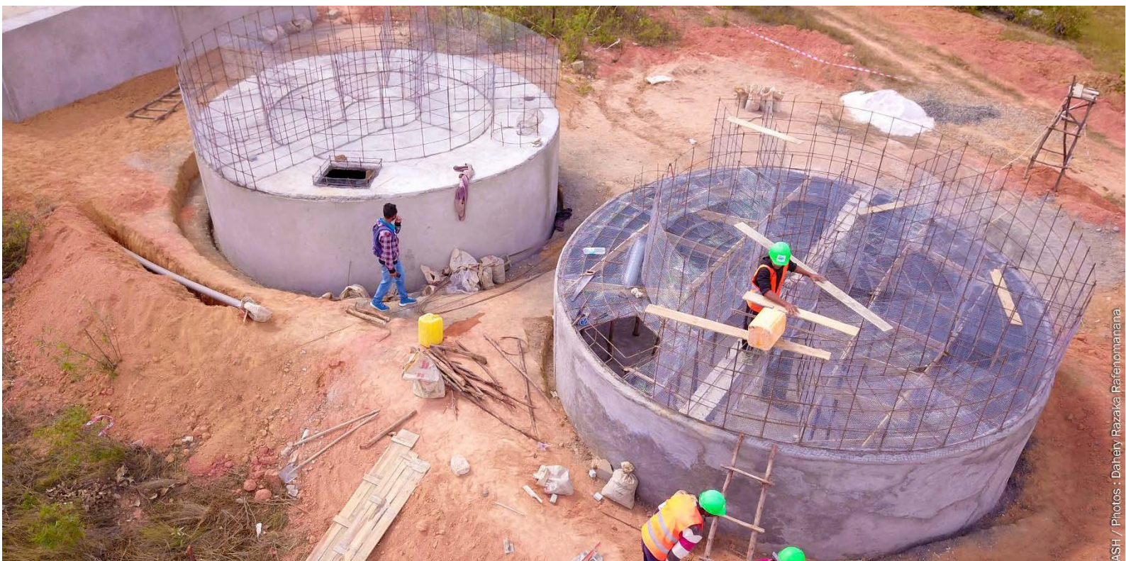
Picture 1. Morarano Chrome (Alaotra Mangoro) construction site. The gravity water supply is equipped with a treatment site with an existing 100m 3 tank and two new 50m 3 tanks. Phot credit RANO WASH
