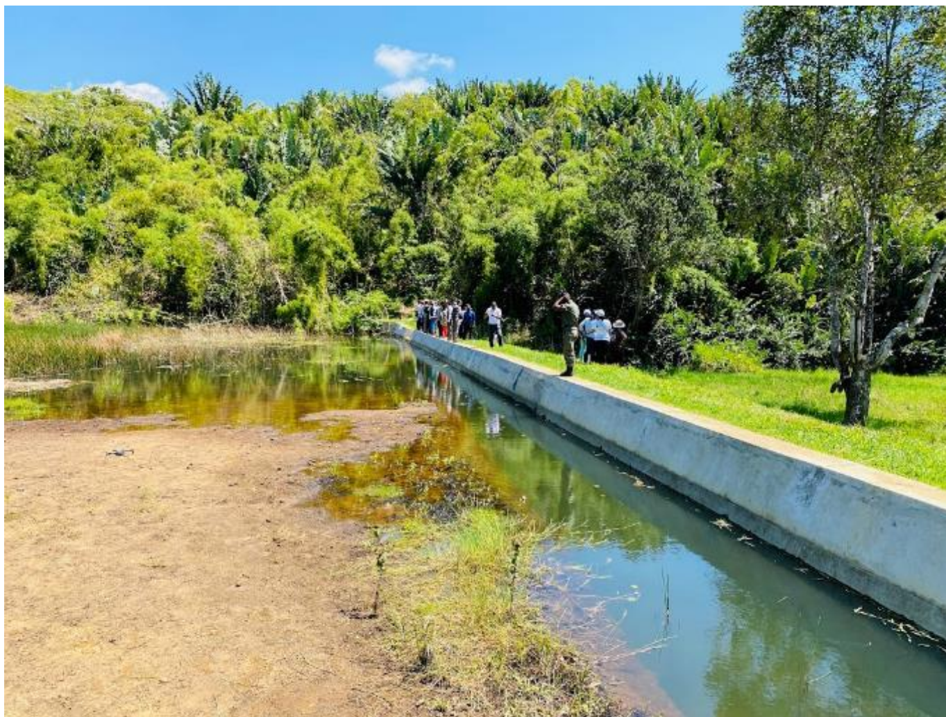
Figure 2: Hillside reservoir in Niarovana Caroline
