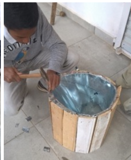
Securing the funnel onto the support. Each tab was trimmed and hammered. (photo credit RANO WASH)
