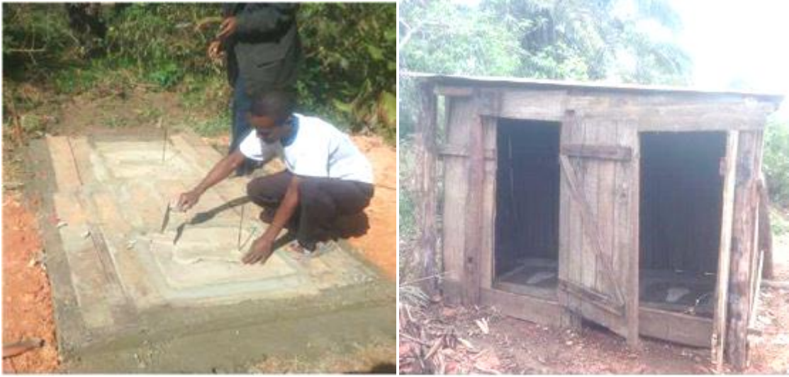
Local builder constructing a hygienic latrine for Amboanjo Primary School.
