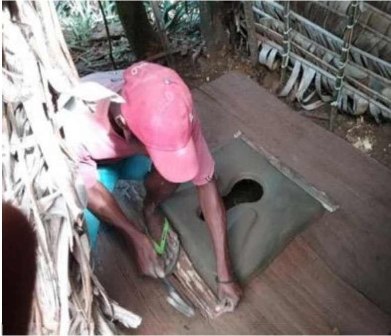
Local mason installing a SanPlat slab
