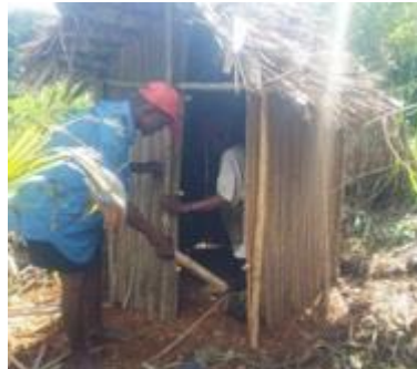
Installation of the walls with a member of the WASH Committee
