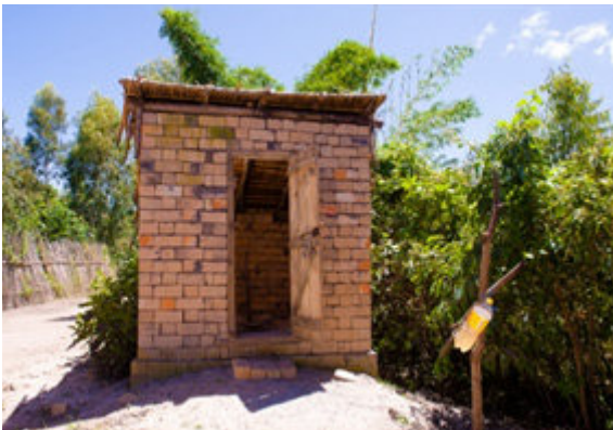
Latrine built by the inhabitants of Ambohimilamina
