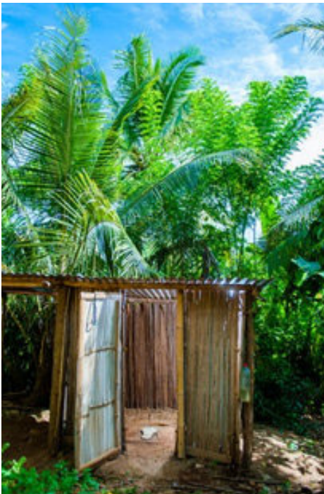
A latrine with san-plat slab installed
