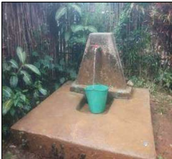
Standpipes rehabilitated through the project
