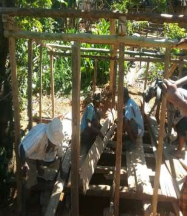
TSABOTO, accompanied by the communities in the construction of his toilet
