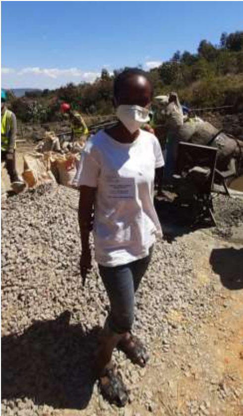
RANOVA HARISOLO Olva Margueritte, 28 years old, young team leader supply in the water system construction, Mickael enterprise in the Commune Androy, Haute Matsiatra region.
