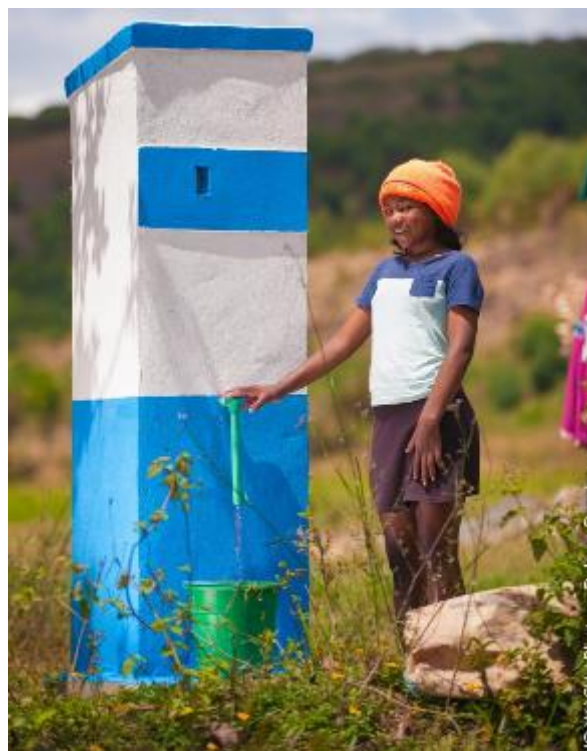
Picture 1. Automatic water kiosk available 24 hours a day created and installed Manampy Corp in the Alaotra Mangoro region
